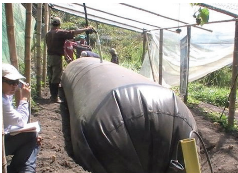
PICTURE TOP: Continuous flow bio-digester installed at Fidel Migue's farm in the settlement of Peñaranda, Ibagué – Tolima. 20 families benefited from the system. Photo Credit AngloGold Ashanti
